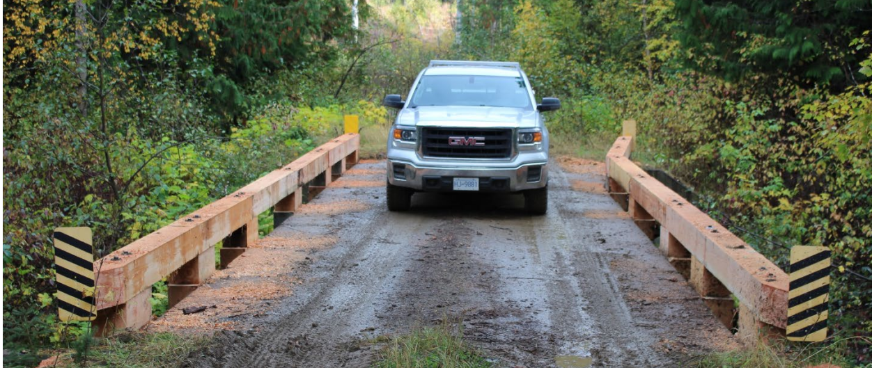
LNTCF SAWMILL CUT TIMBERS FOR BRIDGE REPAIR
