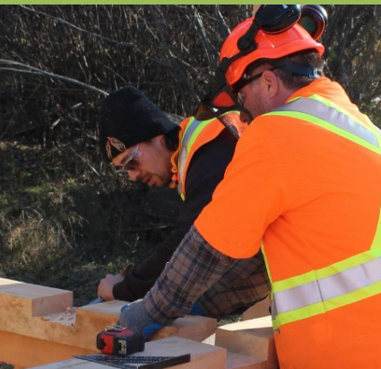
JCP CREW AT WORK LNTCF
