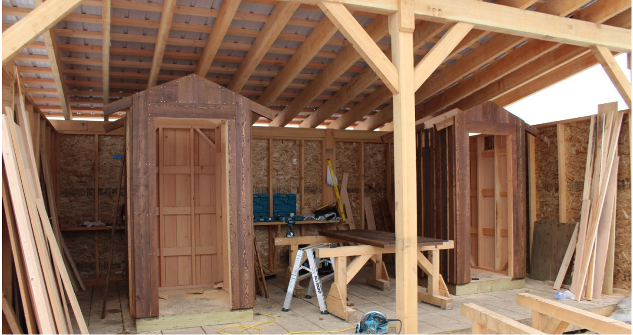
BUILDING OUTHOUSES AT LNTCF
