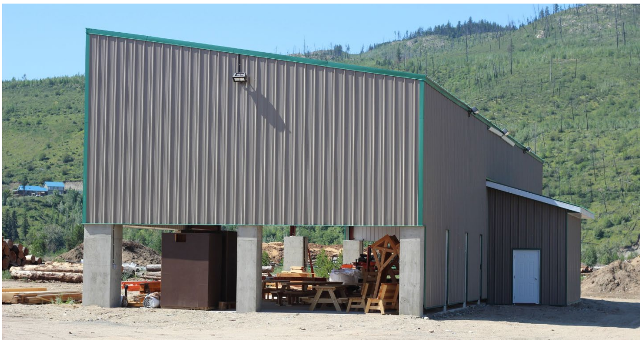
LOWER NORTH THOMPSON COMMUNITY FOREST SOCIETY – MILL BUILDING
